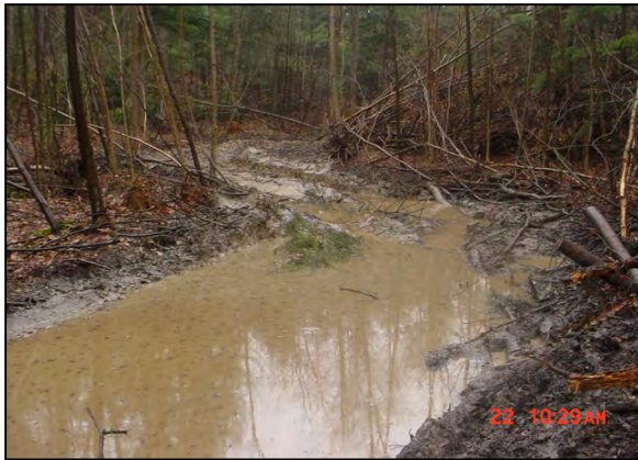
Improperly constructed logging road with poor drainage allows water to collect and sediment to enter the nearby stream.
