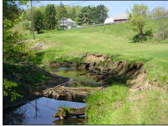
Erosion of streambank due to stream encroachment and poor streamside vegetation
